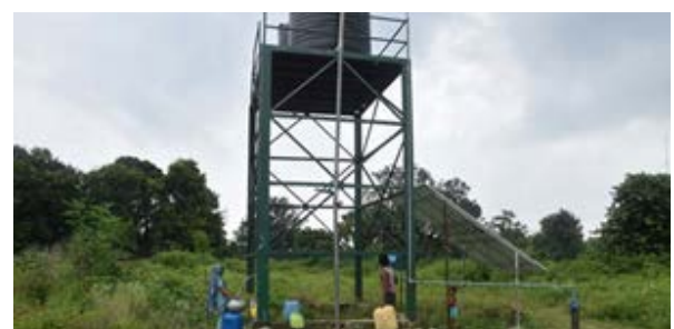
The overhead water tank in the Bhiknathodi village under the 'Har Ghar Nal Ka Jal'
