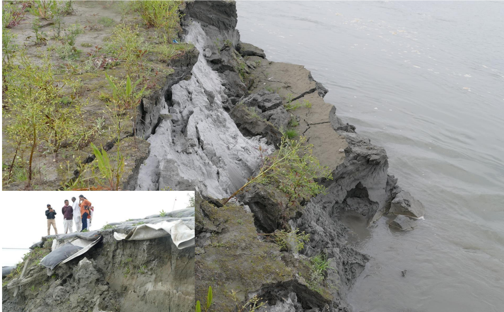
Photo 1: Erosion is the most imminent threat to the existence of the Salmora area as well as the Majuli Island itself. Geobags, being laid now have not been installed properly in some places as per community opinion.
