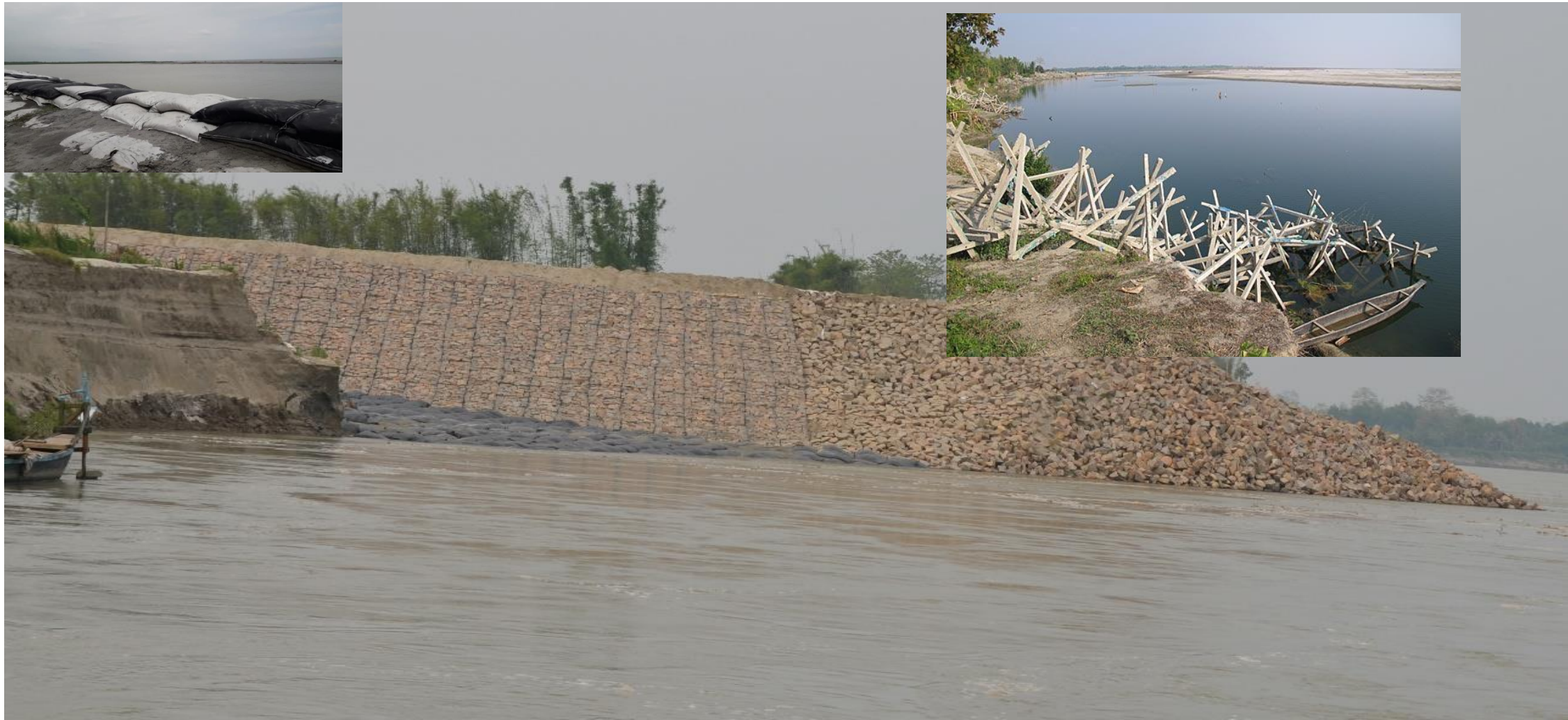
Photo 2: Structural mitigation measures taken by the State and Central Government include use of RCC porcupines to recover land by inducing siltation; Boulder Spur to push an intruding active channel of the river away from a particular stretch of the river bank and geo-bags to resist erosion of river banks. Although porcupines have worked well, the spurs didn't help Salmora area. Success of Geo bags could be limited as seen during the flood of 2019.
