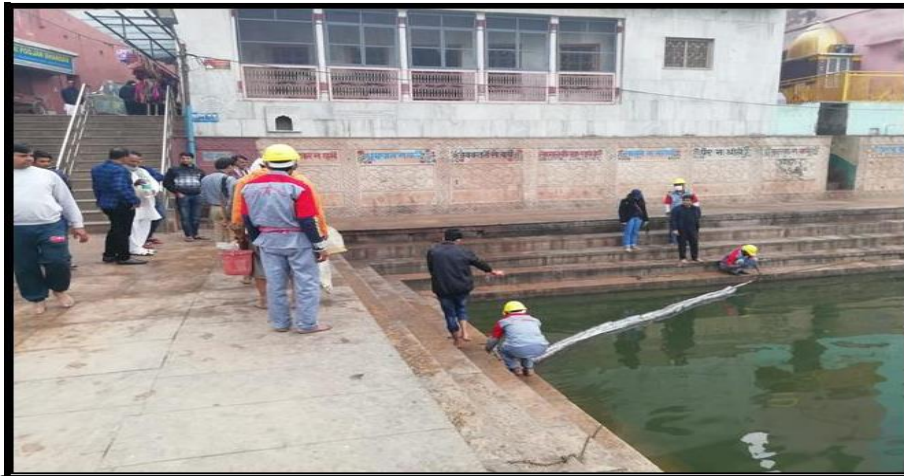
Installation of Bio-fence
