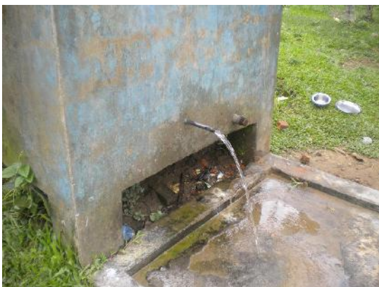
P 13: School Water Tank in Sommeffre village
