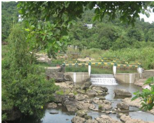
P 16: Check dam at the fish sanctuary
