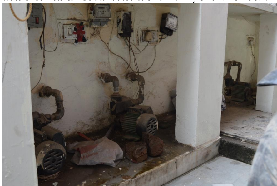
Photo 4: Three pumps being used for pumping water
