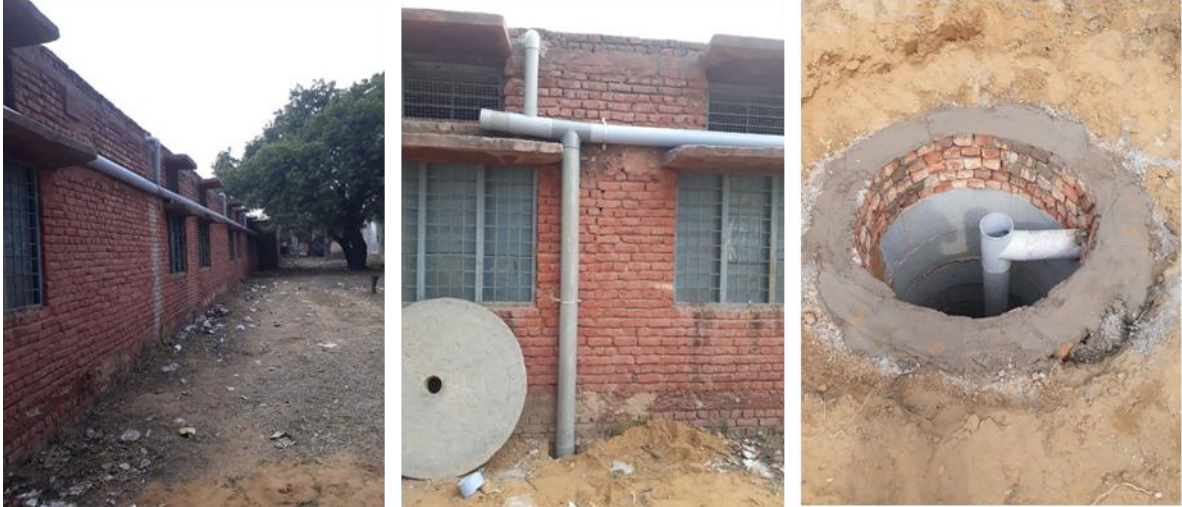
Site images of RWH structure construction
