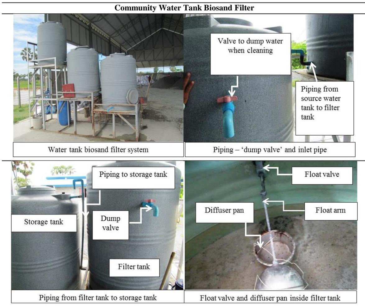
Plastic water tanks are available in most of the cities. They are light to transport, when empty, and generally last for 7 – 10 years. They are inexpensive relative to other container materials and simple to fit
