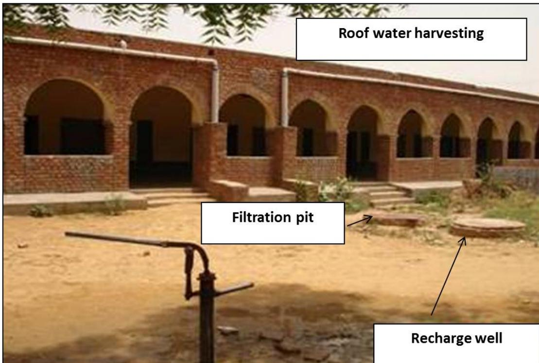
The components of the rooftop rain water harvesting mechanism are:
