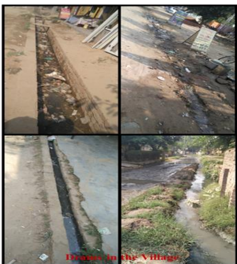
Exhibit 11: Glimpses of waste water infrastructure across the village
