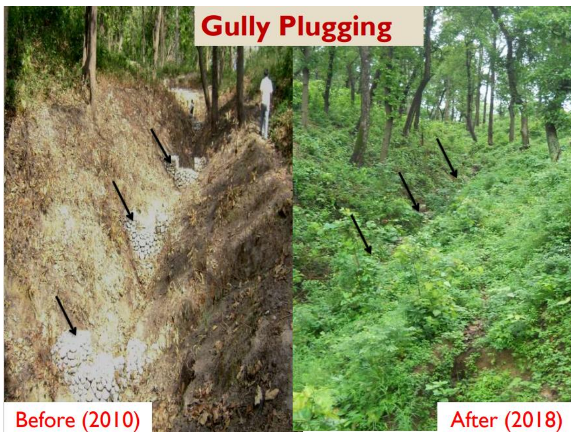
Image 6: Gully plugging undertaken in 2010 and its effect in 2018
