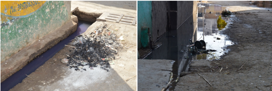
Waste Water on the Roads
