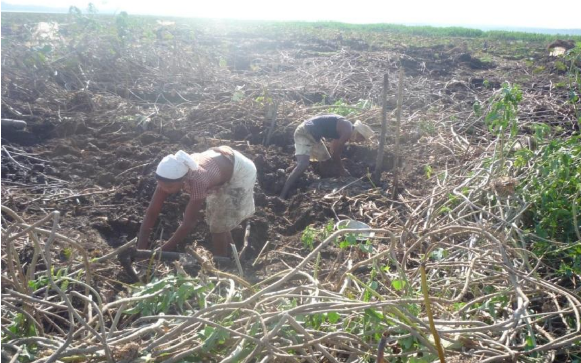
Tank restoration/part-desilting in progress
