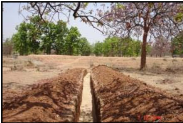
Separate Inlet for diversion of water spillway
