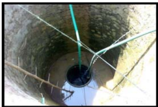
Irrigation well pump
