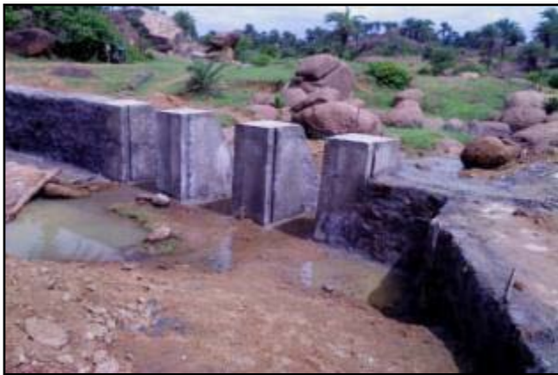
Check dam under construction check dam
